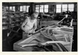
The range of trades incorporated into the Annandale factory was astonishing and the craftsmanship second to none. Frames were hand strung with minute attention to coil spacing and string angle.
